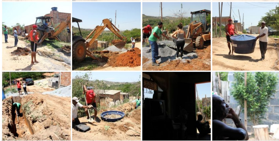
Figure 4 - Construction of the Evapotranspiration Tanks
