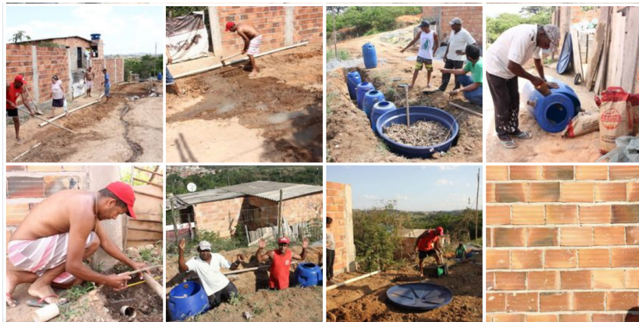
Figure 5 - Construction of the Evapotranspiration Tanks
